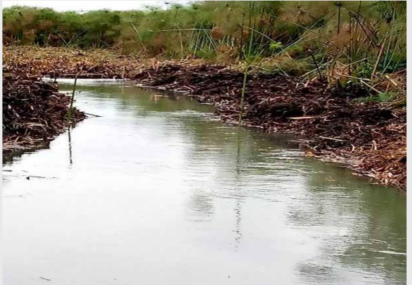
Site clearing in progress.
